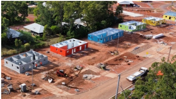
New homes under construction in Yirrkala (NT)
