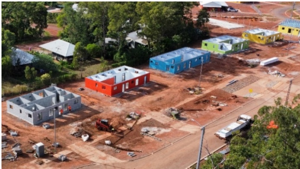
New homes under construction in Yirrkala (NT)
